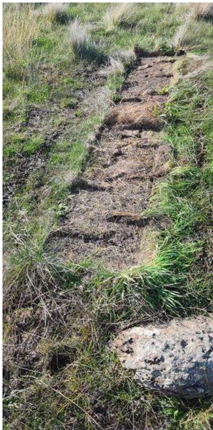
An old trough site about to be repaired
