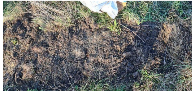
Trough site being repaired
